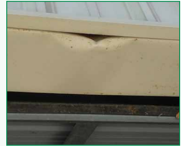
'Door Damage' is from my first week at Hudson, still there after 30 years (left my mark on Hudson Pump!)
